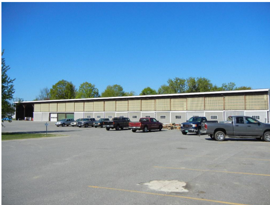
ABOVE IS ANOTHER VIEW OF THE 18 DOOR STORAGE FACILITY WITH AN UPPER DECK JUST TO THE LEFT OF THE MAIN FACILITY WITH 2 OPEN BAYS AT THE END OF THE BUILDING
