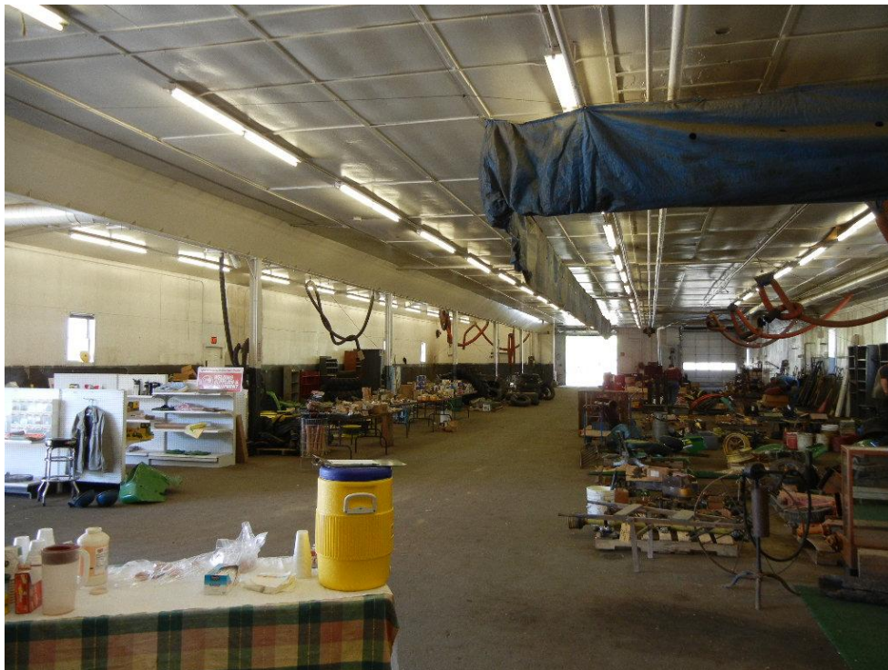
PICTURED ABOVE IS THE SHOP WITH 3 OVERHEAD DOORS LARGE ENOUGH TO ACCOMMODATE LARGE TRAILER TRACTOR UNITS
